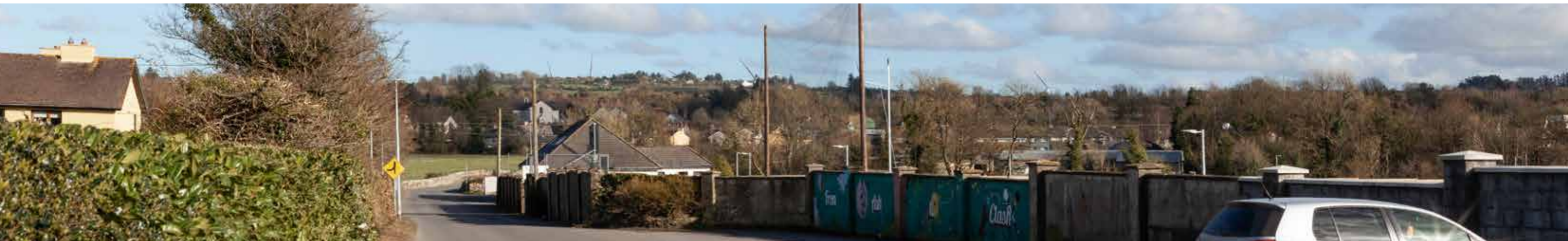
View from the L3423 north of Mullinavat GAA Club of the proposed Ballyfasy Wind Farm
